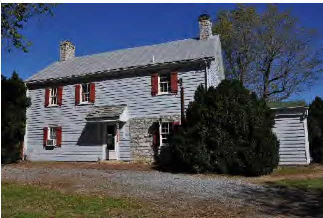
South side of house looking NW (130)
